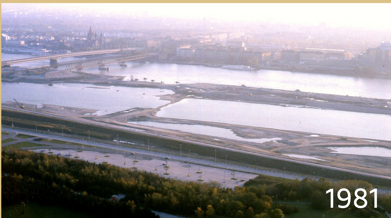
Excavation of the New Danube close to the Reichsbrücke, then a temporary bridge after the collapse in 1976.
