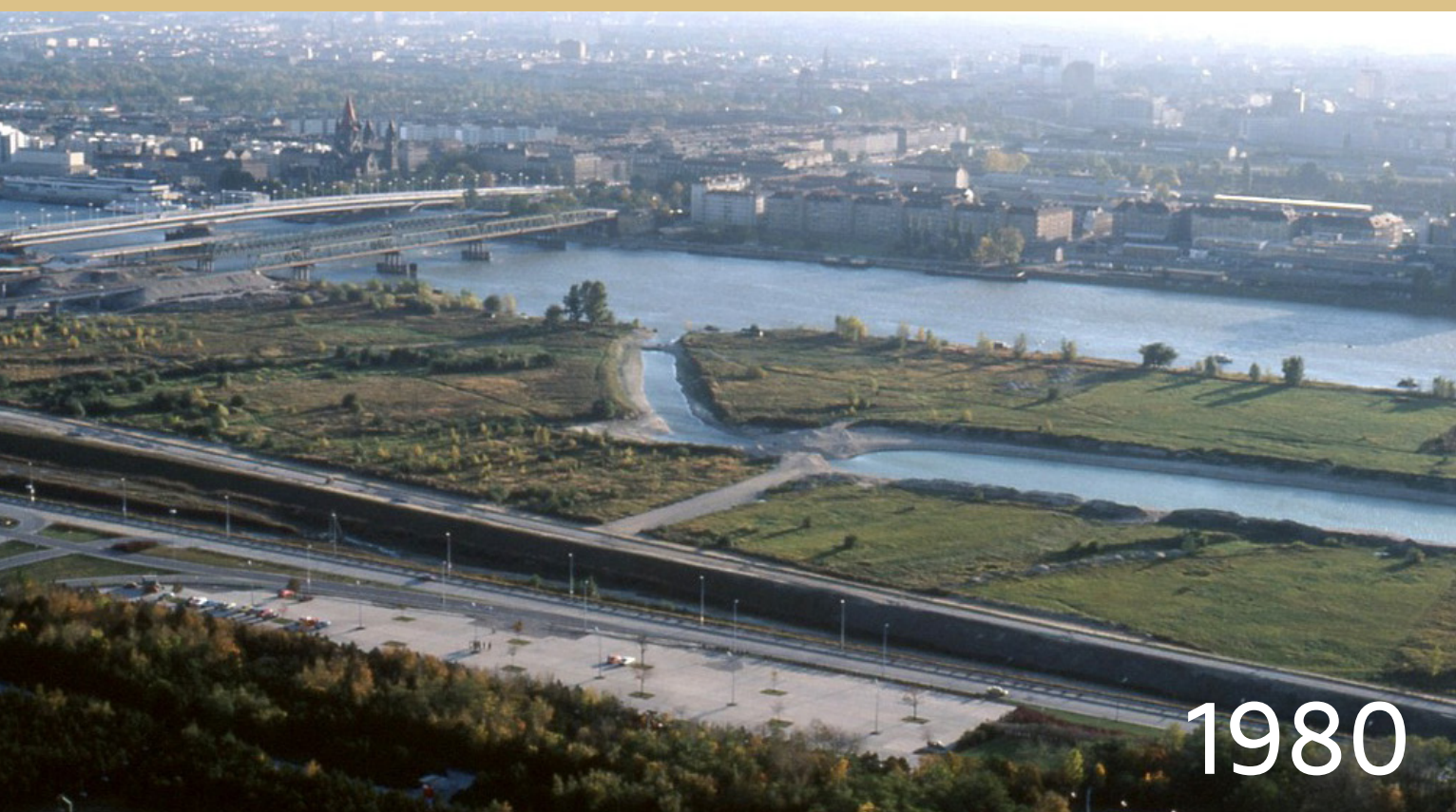
Excavation of the New Danube close to the Reichsbrücke, then a temporary bridge after the collapse in 1976.
